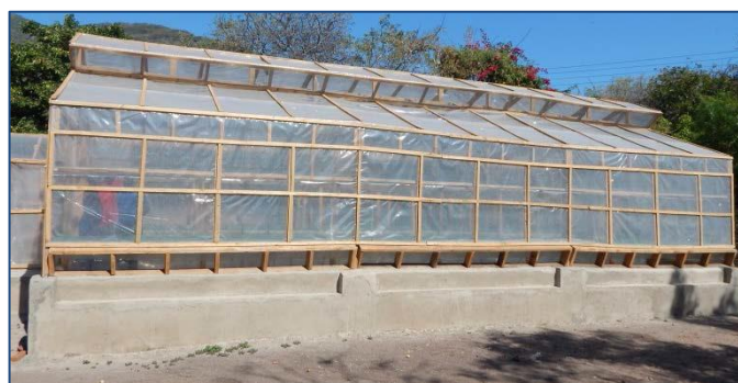
Photo 2. Solar fish dryers are house-like structures with clear UV resistant polythene plastic and venting for air circulation. The size is about 12 x 5 meters.
