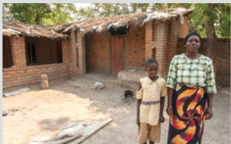
Margaret and her son Shalif outside their thatched home in Vethiwa village, GVH Chipolonga, Machinga. Part of their home was destroyed by torrential rains in January. Through VSL, Margaret is hoping to buy iron sheets to reroof it.
