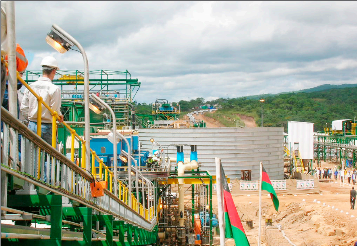
The Kayelekera Uranium Mine puts to test issues of the environment in Malawi especially with regard to energy generation; The mine's generators consume an estimated 800,000 litres of diesel in a month
